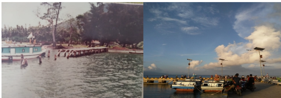
Figures 3a, 3b - The pier on Sebesi Island has long been a vital facility for facilitating population mobility. The pier during the 1980s(left) and during 2022 (right). (Source: authors' collections.)
