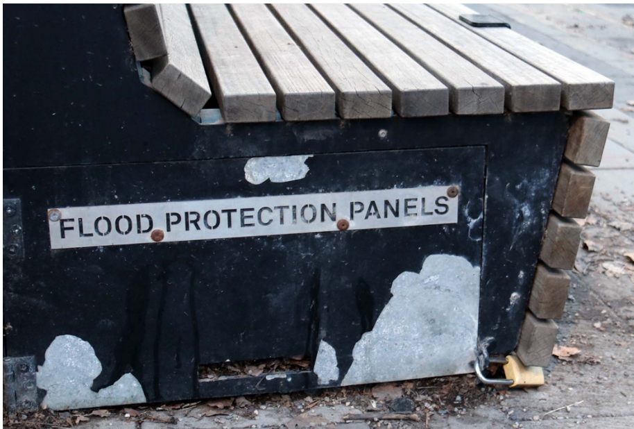
Figure 5 – The wall has gaps for access, with gap-filling panels locked underneath the benches. The presumption is that a flood warning leaves time to find the key, unlock the storage area, and slot in the panels (2024).
