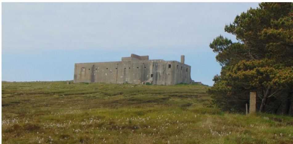
Figure 9 - The now abandoned radio control centre located on a hillside outside of Lyness (author’s photo 2018).
