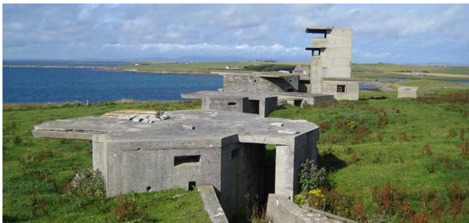
Figure 13 - Former military sea defences at Hoxa Head on the island of South Ronaldsay, which guarded the main southern entrance to Scape Flow (author's photo 2016).
