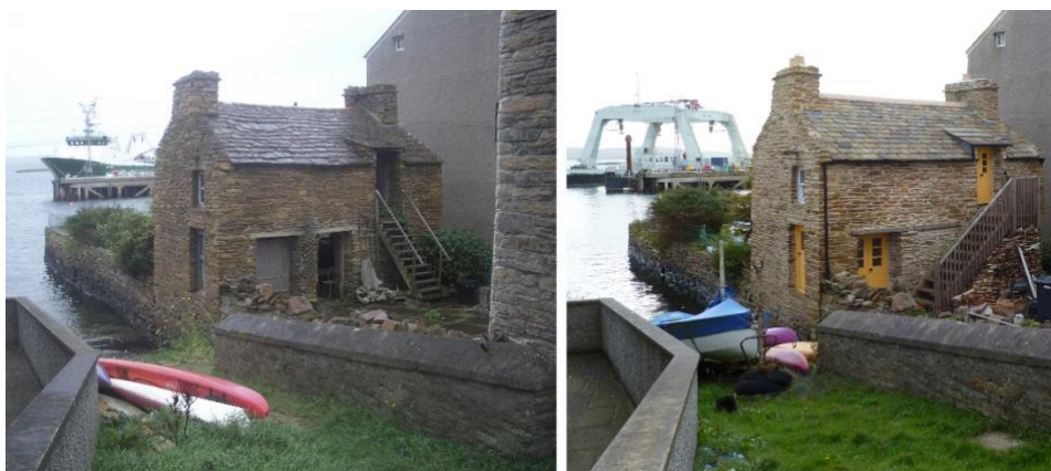
Figure 6 - A comparative view of building renovations in Stromness, also indicating the transition from fishing to service vessels, alongside scaling up of marine activity, in the background (author's photos 2012, 2020)
