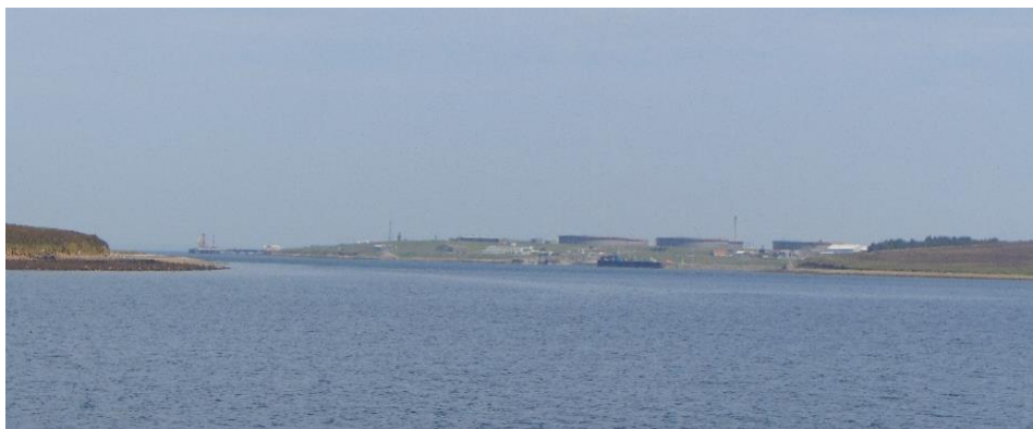
Figure 12 - View from Lyness to the Flotta Oil Terminal. The flare stack is less noticeable in daylight, but just visible to the right side of the terminal (author's photo 2023).
