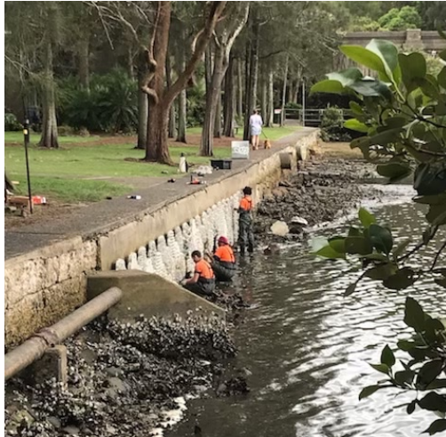
Figure 2 – Installation of marine panels on Burns Bay embankment (January 2024, author’s photo).
