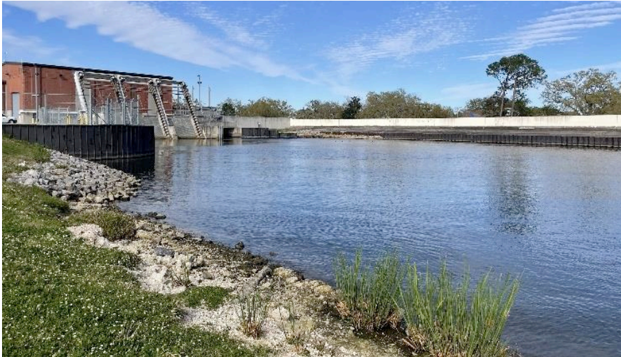
Figure 8 - Floodgates at the northern end of BSJ (photo by Mallum, 2022).
