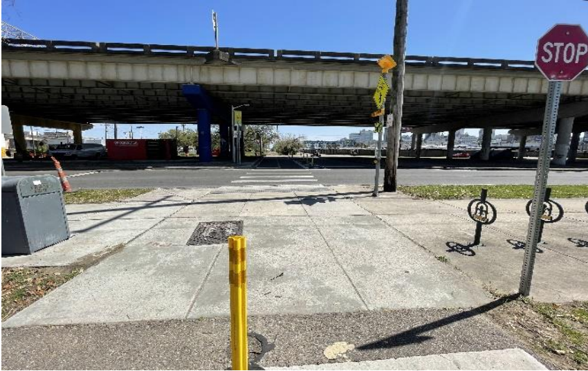
Figure 17 - Elevated section of Clairborne Expressway (photo by Mallum, 2022).
