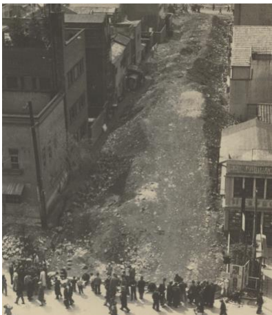
Photos 1 & 2 - Ryukangawa in 1948 and being reclaimed in 1949 (Courtesy of Chuo City Library).
