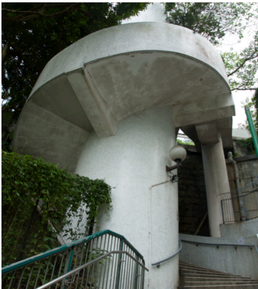
Figure 23 - Spiral staircase (2017, author's photo).
