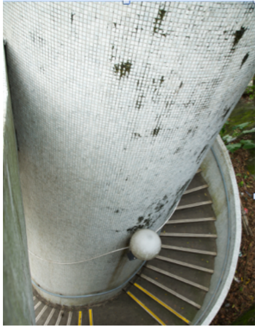
Figure 27 - Spiral staircase (viewed from top) (2017, author's photo).
