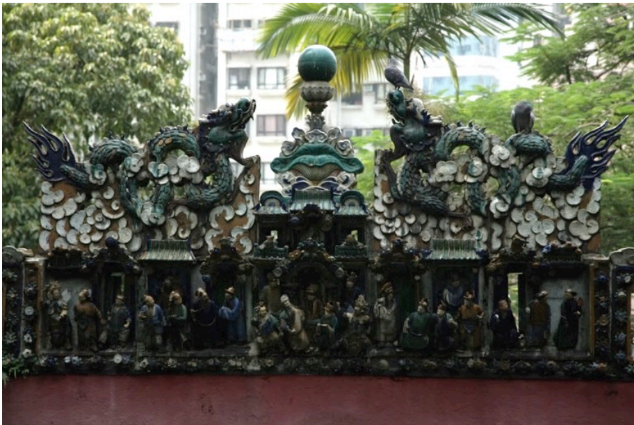
Figure 25 - A Close-up of Lo Pan Temple's Rooftop (2017, author's photo).
