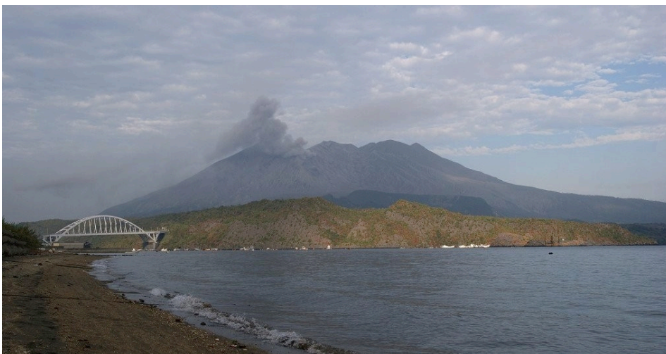
Figure 6. Ushine Ōhashi (bridge) between Sakurajima and the Ōsumi Peninsula. (Courtesy of PhotoMiyazaki(MORIMORI), http://kagoshima.pmiyazaki.com/sakurajima/o2_ushine_br.htm - accessed 1 March 2014).
